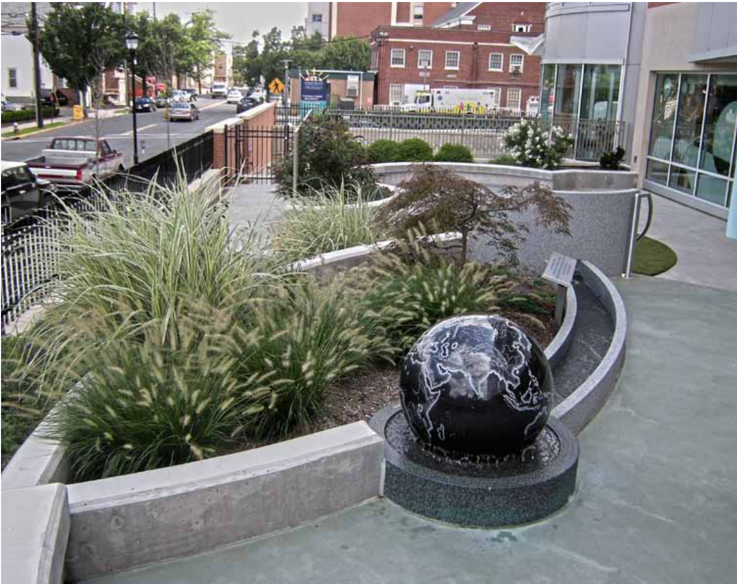
A curved, about 13' long granite runnel connects the Ø 2' 6" Floating sphere to the Ø 7' granite fishpond. The Floating sphere fountain, runnel, and fishpond were prefabricated and tested in Kusser's plant in Germany before shipping.
